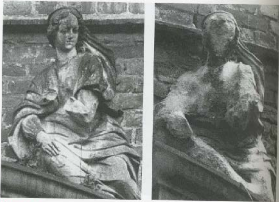
Figure 10.6. Sandstone figure over the portal of a castle, built in 1702, in Westphalia, Germany, photographed in 1908 (left) and in 1968 (right). The erosion of the figure is due to a combination of acid deposition and air pollution produced from the industrialized Ruhr region of Germany. Courtesy Horv Schmidt-Thomsen.
